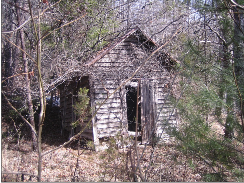
Photo 9. Shed A, view northeast.
