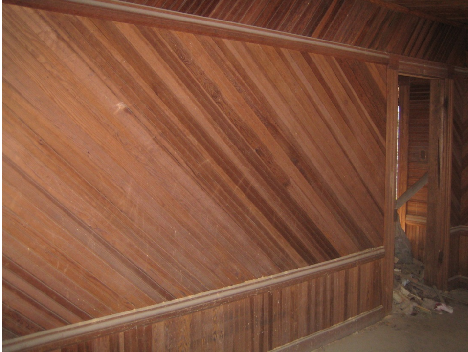
Photo 6. House, west room of main block, view southeast. The doorway accesses the center hall; the door frame of the main entrance is just visible through the doorway.
