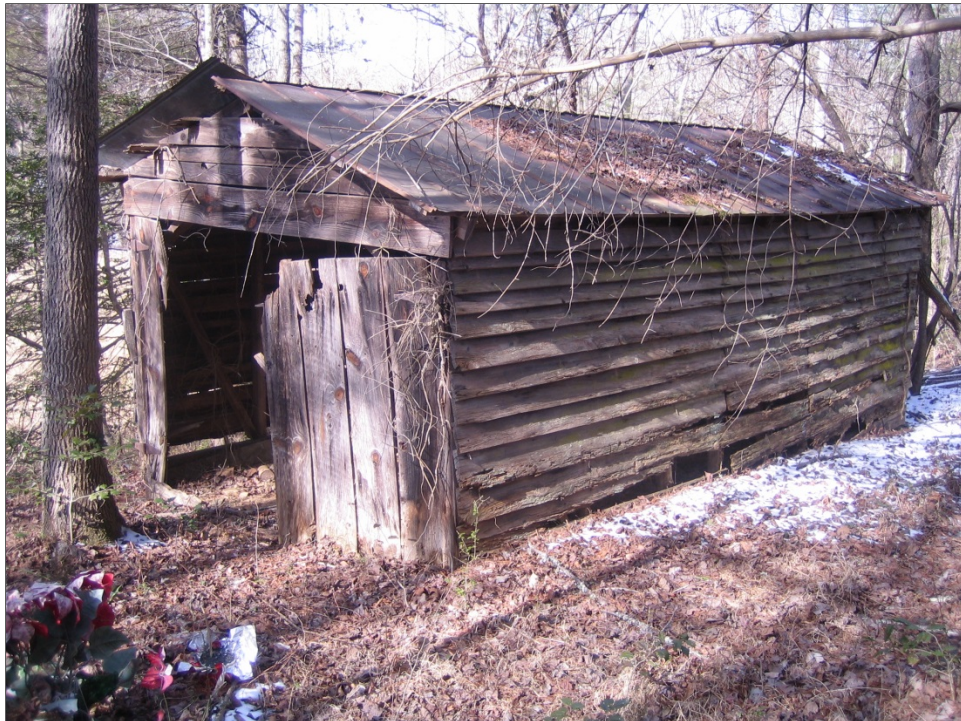
Photo 20. Shed B, view southwest.
