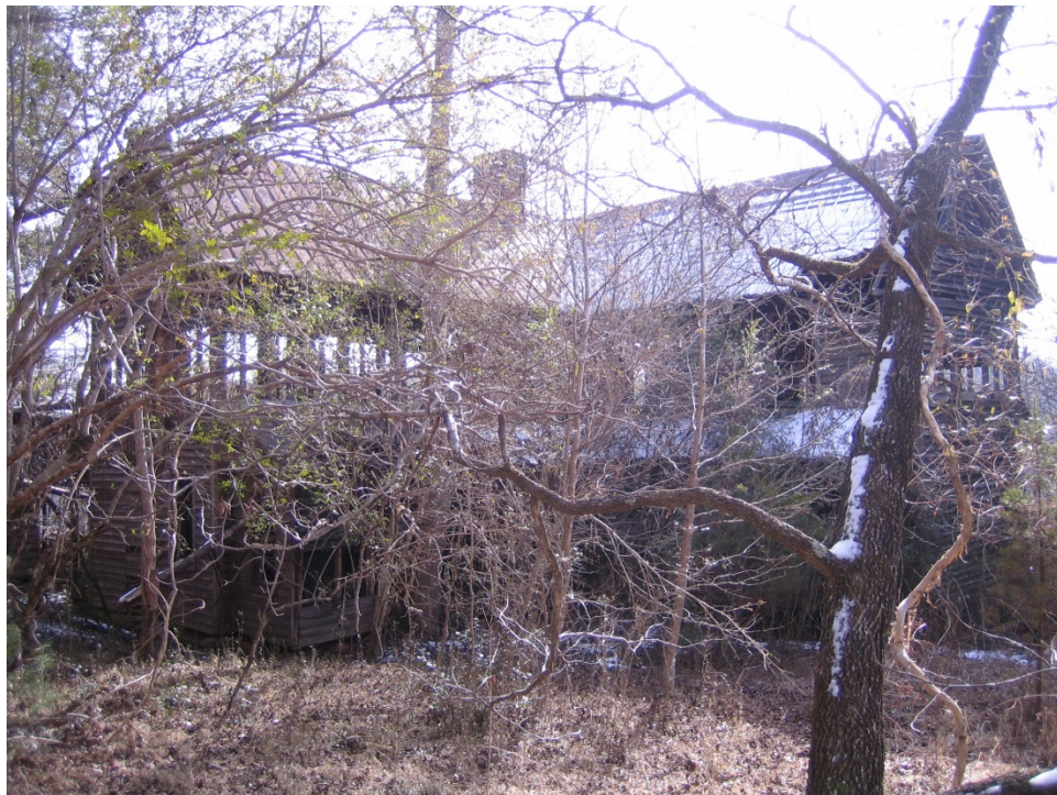
Photo 5. House, rear ell and rear of main block, view southeast. Note the missing weatherboard at the second story. Much of the weatherboard is missing at the second story of the rear ell.
